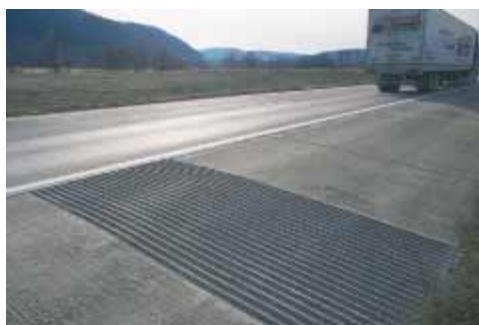
Figure 18.13 Rumble strips along the side of a highway.
