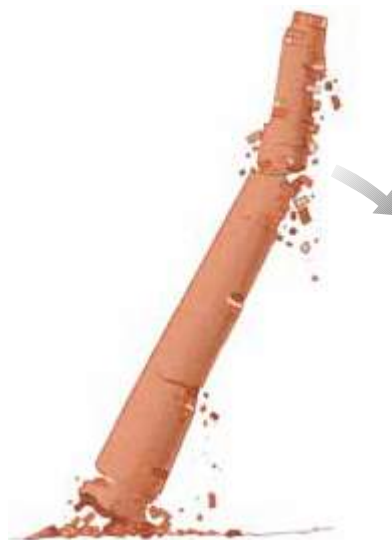
Figure 10.19 A falling smokestack.
