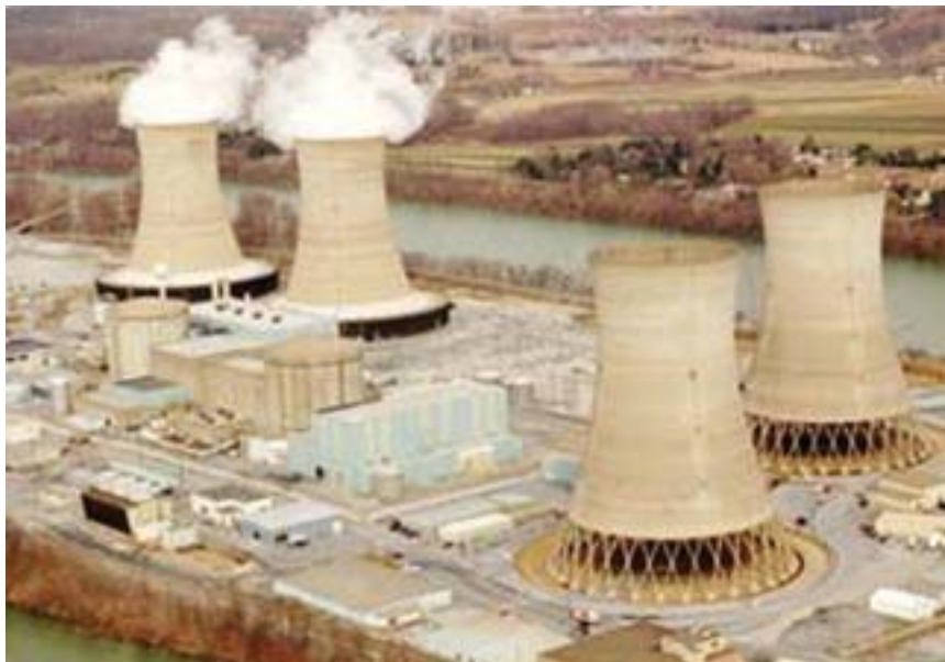
Nuclear Power Station
