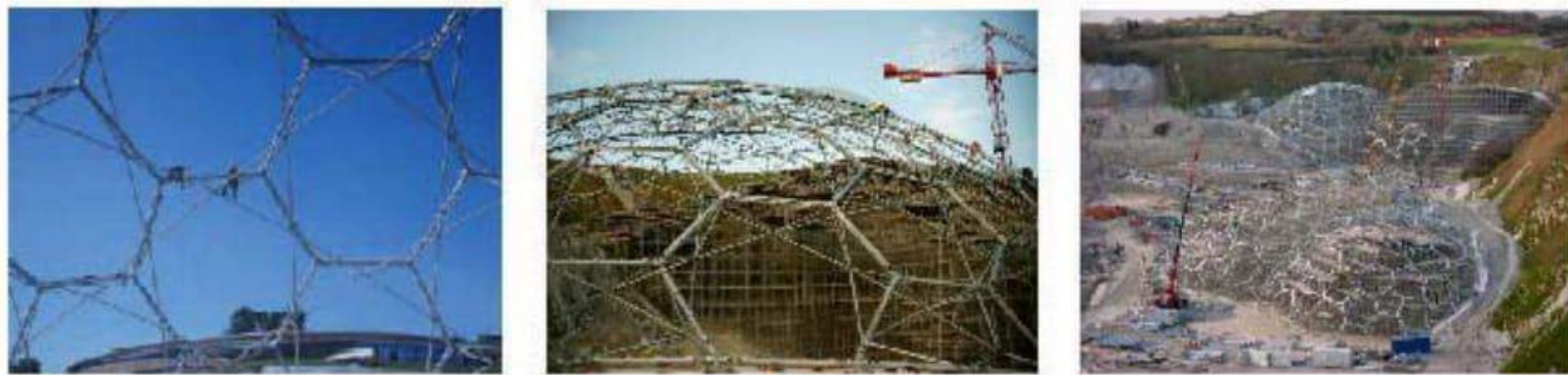
Figs. 39-40. Eden Project, Cornwall, GB, Nicholas Grimshaw Architects, Anthony Hunt Associates engineers, structure: MERO Membrane ETFE-Pillows diameter 9 m, Dimensions: 15 590m 2 , 100m × 220 m height 55 [www.anthonyhuntassociates.co.uk]
