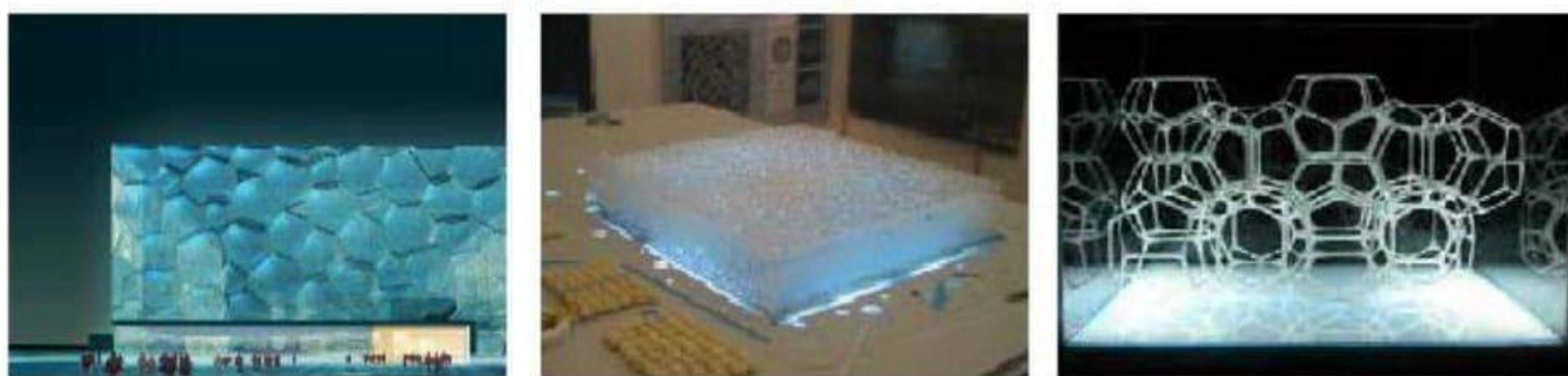
Figs. 44-46. The Rendering, model and structure model shows the three dimensional arrangement of the polyhedral structure, a common natural pattern seen in water bobbles and organic cells. The building envelope acts as an very efficient green house where 90% area. [Ove Arup Pty Ltd, www.ptw.com.au]
