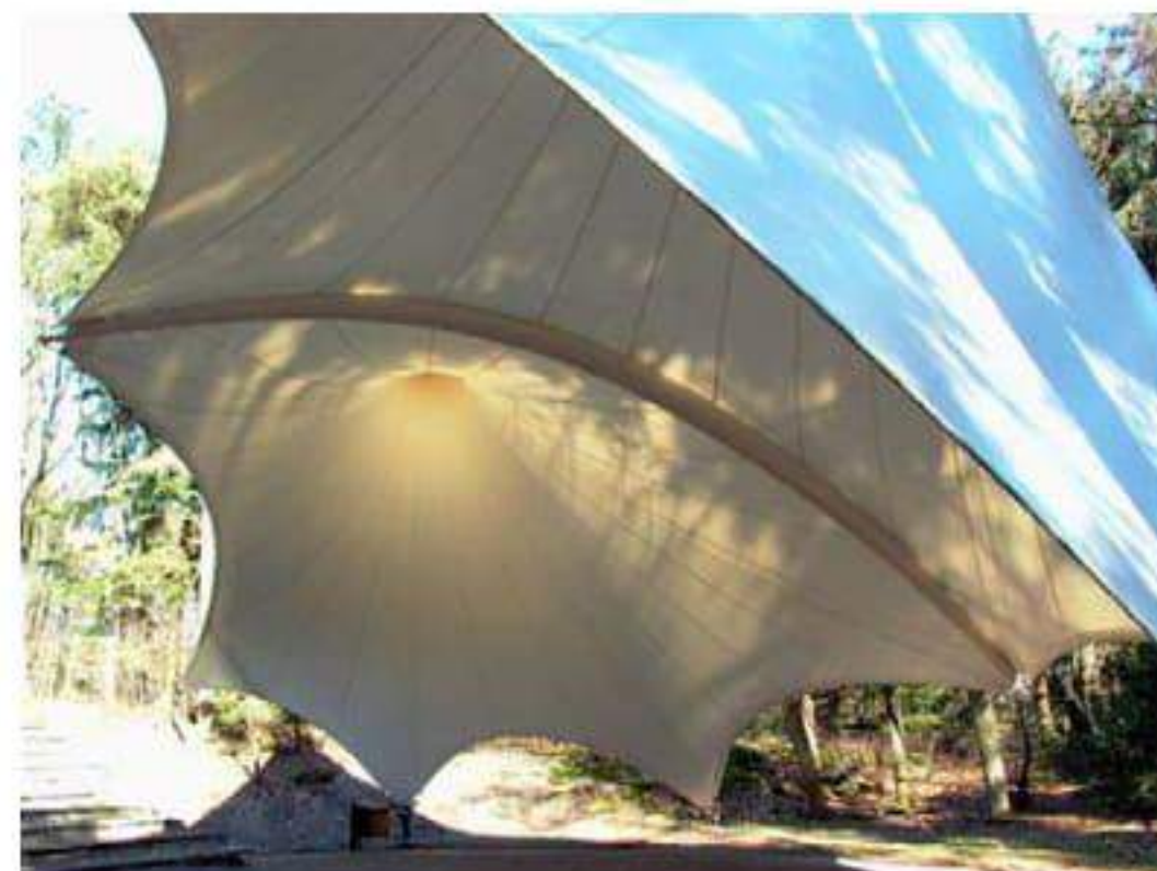
Fig. 8. An arched beam ensures an increase of the protective area and the curvature of the membrane structure
