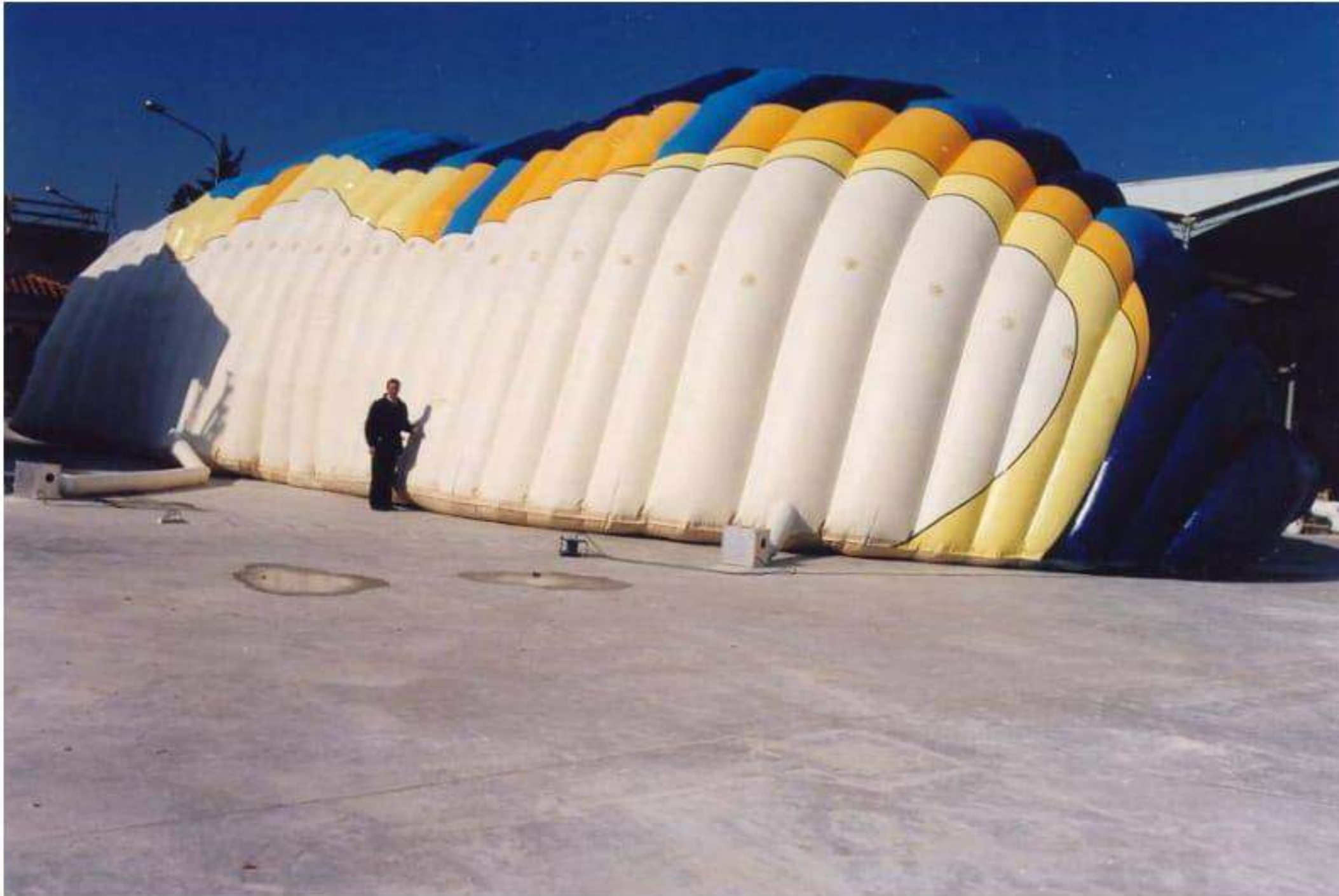
Fig. 4. Inflatable pavilion ( 250\text{m}^2 ) formed by an assembly of low pressure tubes built for the mobile exhibition for the Gaudi Year of Construction Artisans, Barcelona 2002
