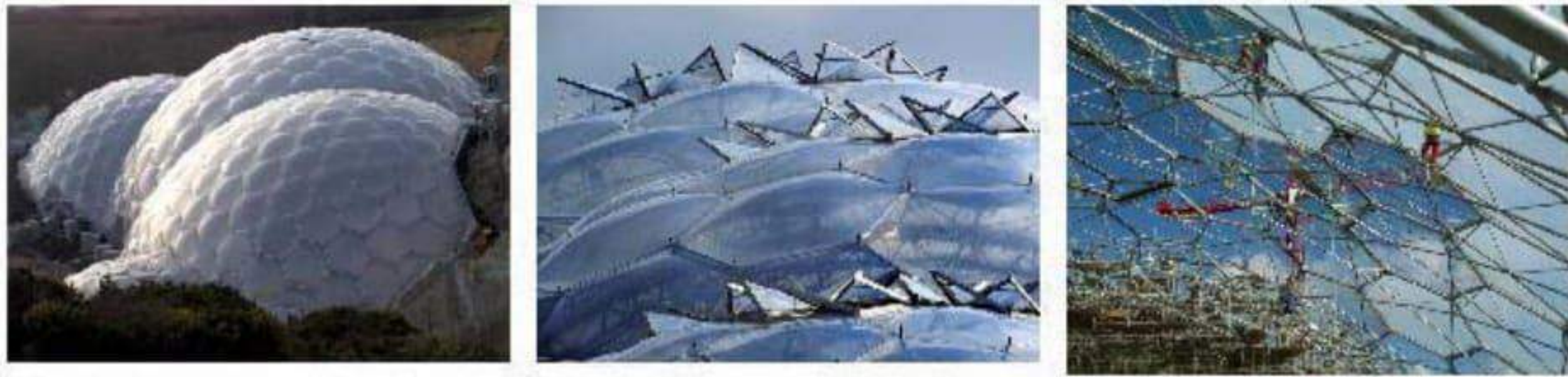
Figs. 41-43. The transparent foil 'windows', made of 3 layers of ETFE (ethylenetetrafluoroethylene-copolymer), form inflated 2-metre-deep pillows. ETFE has a lifespan of over 25 years, transmits UV light, is non-stick, self-cleaning and weighs less than 1/10th the equivalent area of glass and has a great stress redundancy. [www.anthonyhuntassociates.co.uk]
