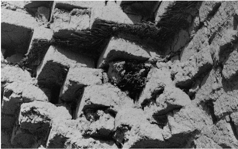
14.7 Woven mat and plaited rope reeds used as reinforcement in the Ziggurat at Dur Kurigatzu.
