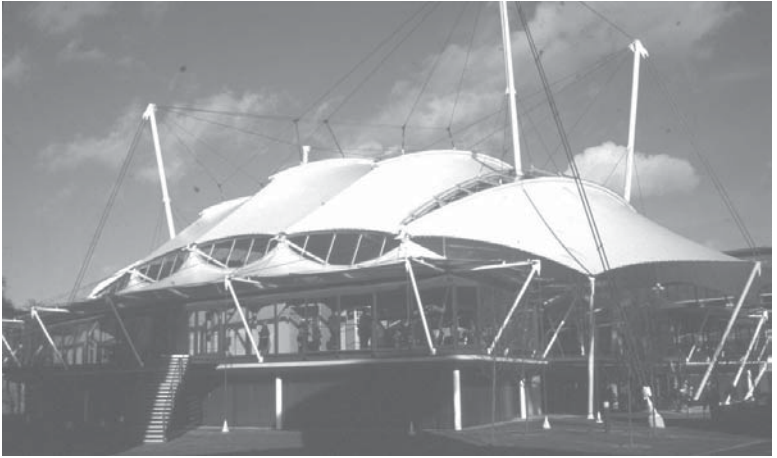
12.6 Membrane roof at the Inland Revenue amenity building, Nottingham, UK (photo: John Chilton).
