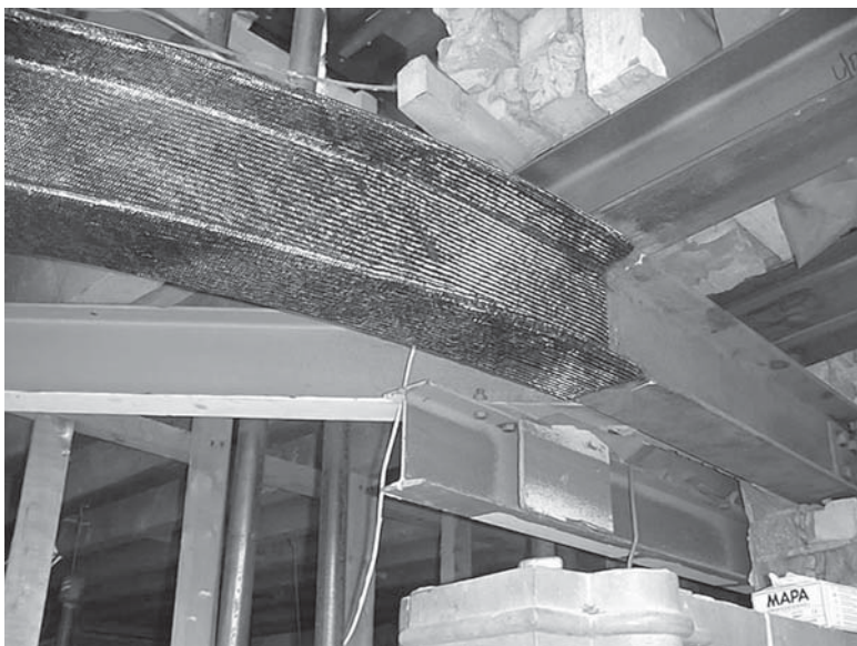
12.4 Placement of a carbon prepreg layer around the flanges and web of a steel beam (photo: Advanced Composites Group Ltd).
