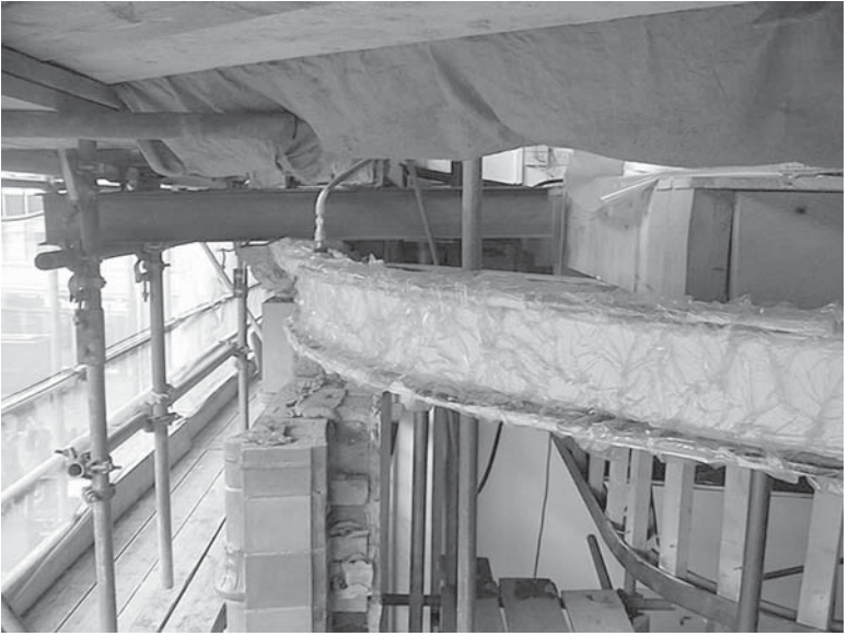
12.5 A vacuum bag used to apply pressure on the composite material (photo: Advanced Composites Group Ltd).
