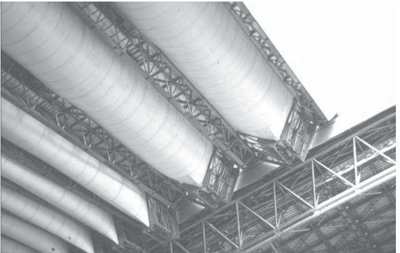
12.2 Synclastic form of the air-inflated membrane tubes for the deployable roof of the Toyota Stadium, Toyota City, Japan (photo: John Chilton).
