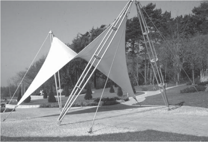
12.1 Simple anticlastic form of a small canopy, Millennium Garden, University of Nottingham, UK. The form has two high and two low points creating a classic saddle surface (photo: John Chilton).
