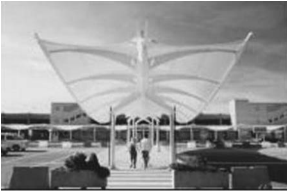
18.23 Entrance and walkway areas architectural membranes [65].
