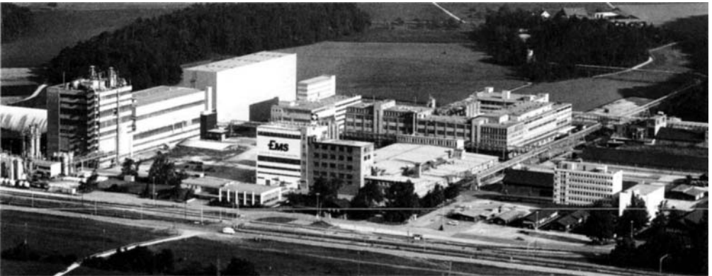
Figure 1.19 Areal view of a complete production plant for polyester and polyamide 6 filaments, staple fibers, chips, synthetic thermo bonders and other specialties. Start of construction around 1950 from a wood saccharisation plant; extended and reconstructed in phases; photo of 1992 [48]
