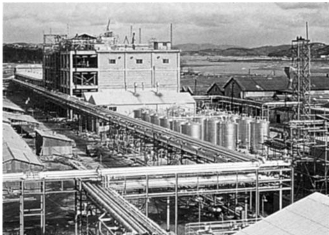
Figure 4.38 Outside storage area of a PET staple fiber plant with integrated continuous polycondensation (Fourné, 1963/64, Japan)
