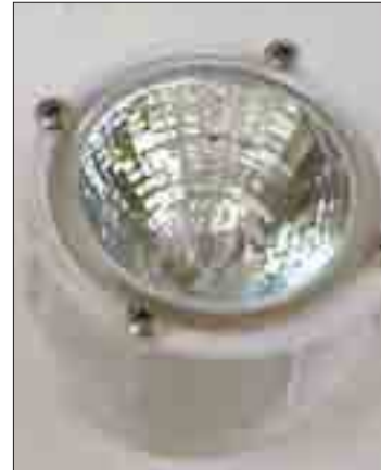
Retaining screws on a lamp.
