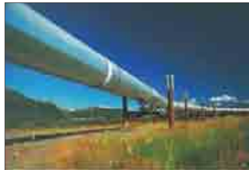
The Trans-Alaska Pipeline carries crude oil 1,284 kilometres through Alaska. The pipeline is 1.2 metres in diameter and can transport 318 million litres of crude oil a day.
