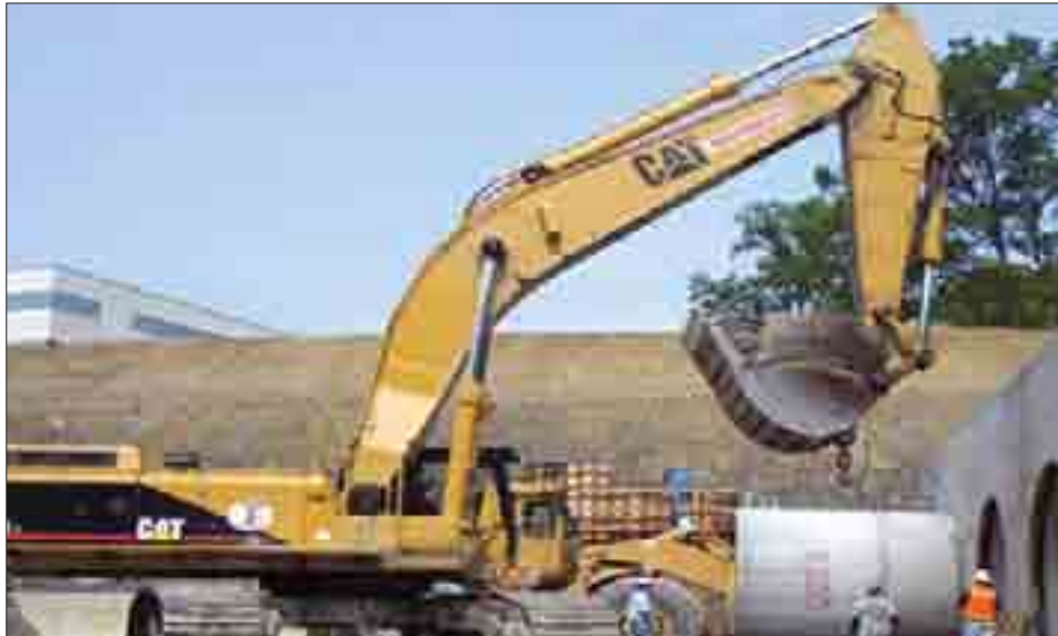
Excavator in action
