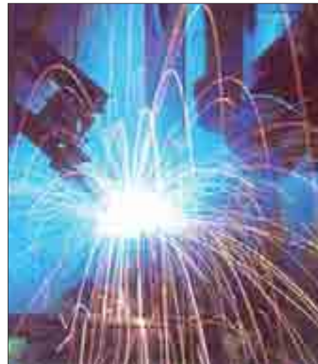
Electric arc welding
