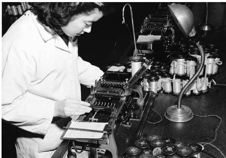
1.12 Testing raw silk for cohesion with a Duplan tester.
