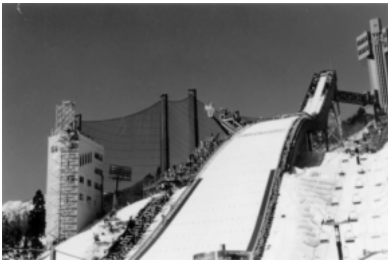
2.18 Wind/snow proof net set near jump shanze at Nagano Olympic Games (Teijin).
