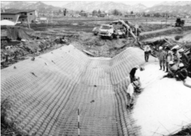
2.19 Construction site using geo-membrane (Teijin).
