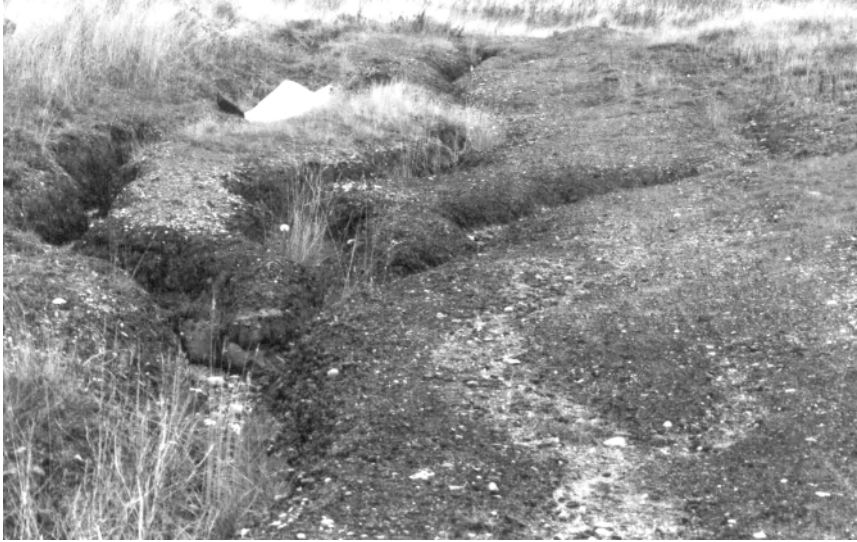
12.9 Eroded surface of a waste tip (note the sparseness of the vegetation).
