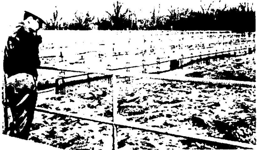
Figure 27-12. An activated-sludge basin with a full load of sewage in the process of aerobic microbiological treatment. (Courtesy of Washington Suburban Sanitary Commission.)
